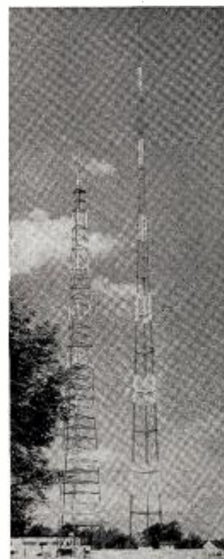
WKBN-TV Truscon Self-Supporting Tower 539-Feet Tall
